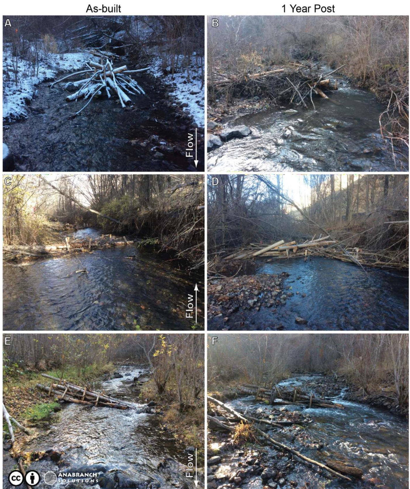
Figure 4. Example of PALS evolution over the course of one year promoting processes of wood accumulation. A and B show a mid-channel PALS becoming a bank-attached PALS, C and D show a bank-attached PALS becoming a debris jam, and E and F show a bank-attached PALS becoming a mid-channel PALS. The geomorphic changes imposed by the presence of the PALS in each example shows clear alterations to the channel bed and hydraulics. From Chapter 4 of Wheaton et al. (2019: http://lowtechpbr.restoration.usu.edu ).
