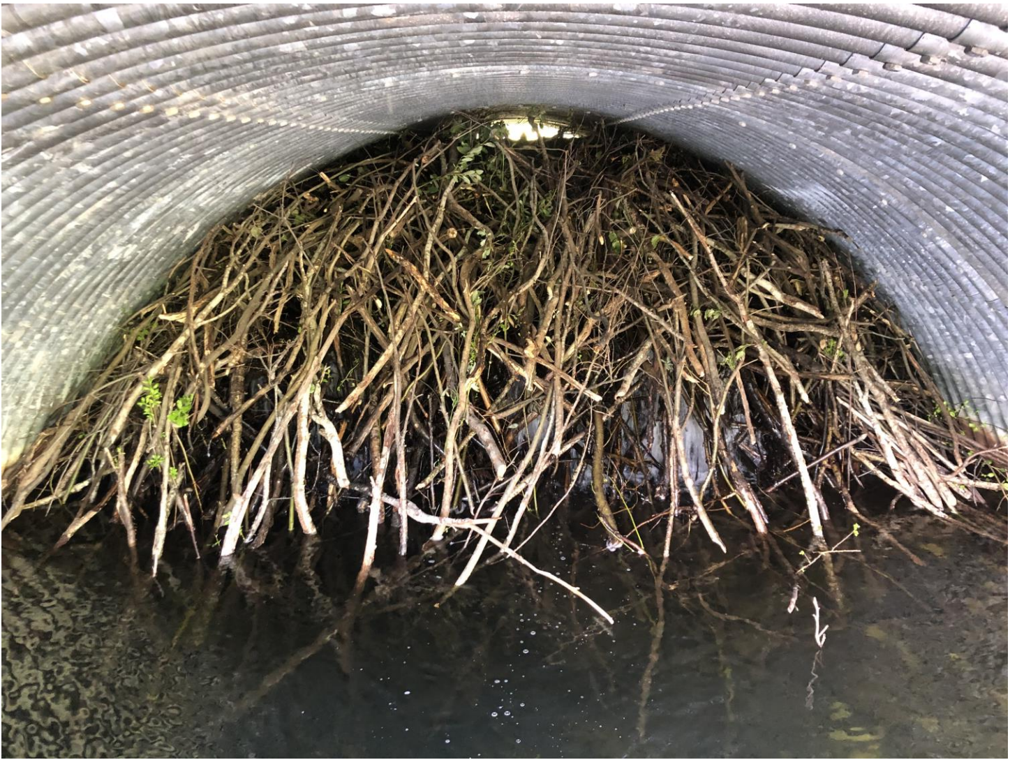
Mill Creek Culvert – Beaver Coexistence
