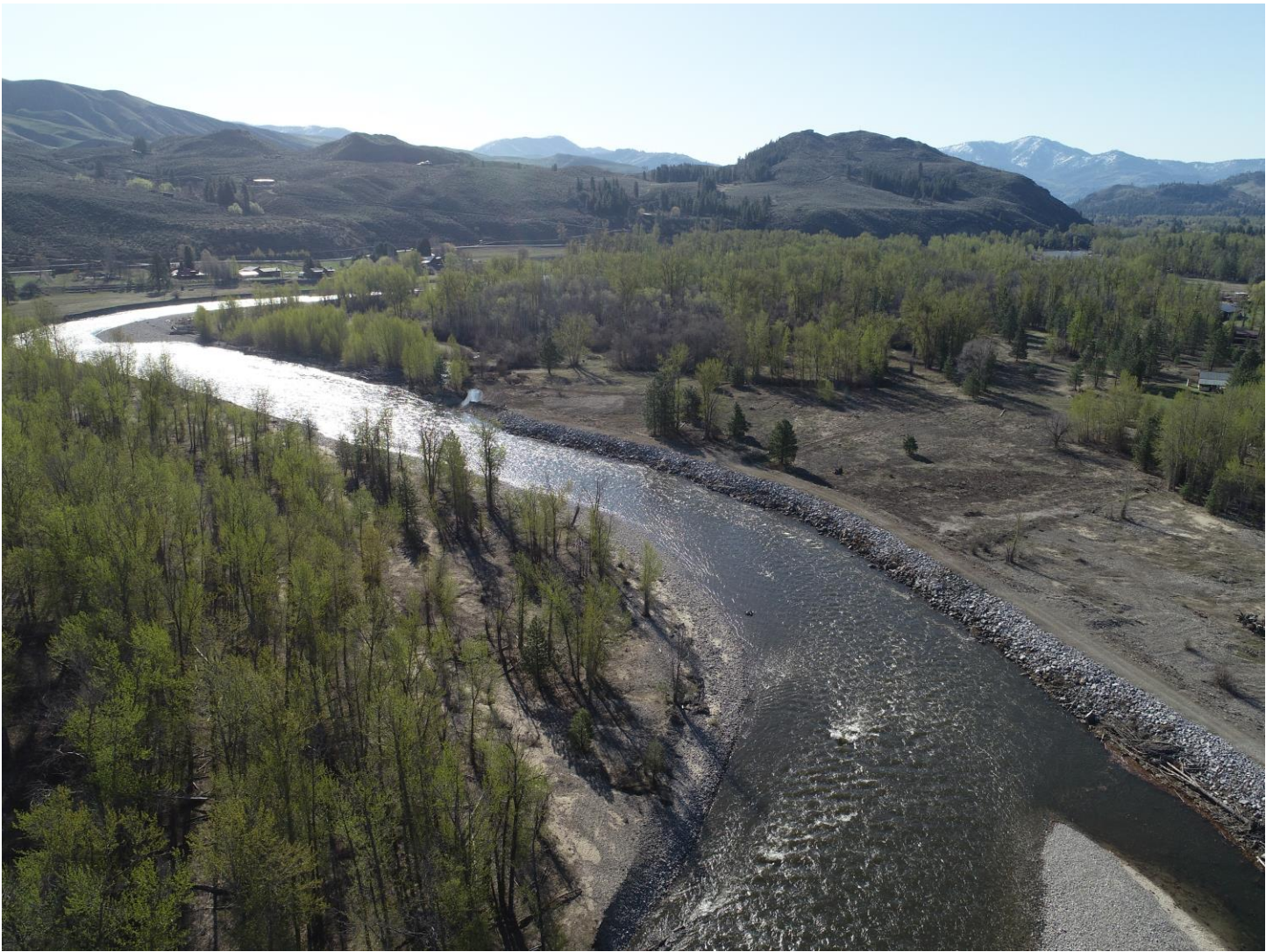
Sugar Right Project Area – levee, floodplain
