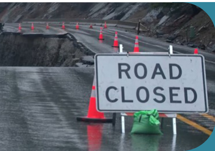
Figure 12: Recent closure of US Highway 5 due to flooding and erosion by the Wenatchee River. (From: King 5 Seattle)
