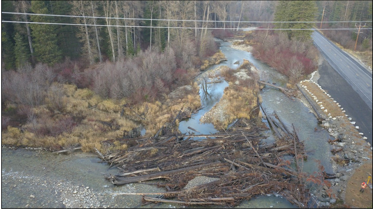
Figure 2. Looking downstream at existing log structure, BPA powerlines, and Highway 207 CED 2 site near RM 4.1. Note riprap placed at right to reduce damage to highway embankment.
