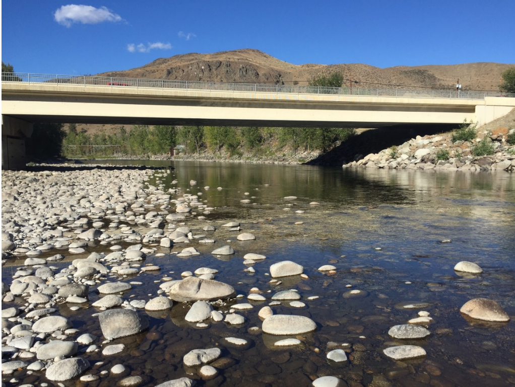
Figure B-6 RM 40.4 – Looking upstream at the Highway 20 bridge crossing. Pebble count data collected at this location in 2016.
