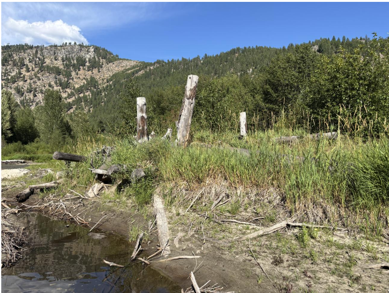
Figure 66. Engineered log structure associated with Dillwater LWD Enhancement project in Segment 3. Structure was originally installed within the Entiat River channel but is now partially buried by sediment on the river left floodplain.
