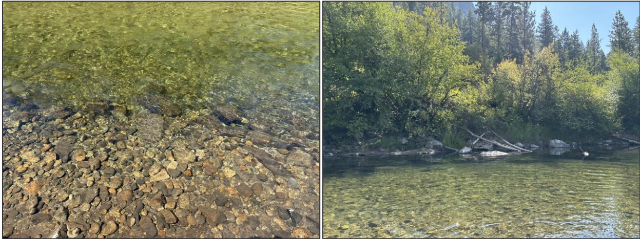
Figure 39. Human alterations in Segment 2. Left: angular small boulders along river left Entiat River channel margin at RM 20.9 are likely remnants of riprap removed as part of Stormy B restoration project. Right: placed boulders along river left channel margin protecting Entiat River road, RM 21.5.
