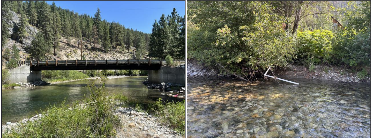
Figure 70. Notable human alterations in Segment 4. Channel spanning bridge crossing the Entiat River at RM 25, looking downstream (left), and PVC pipe extending into Entiat River channel near RM 26.3.
