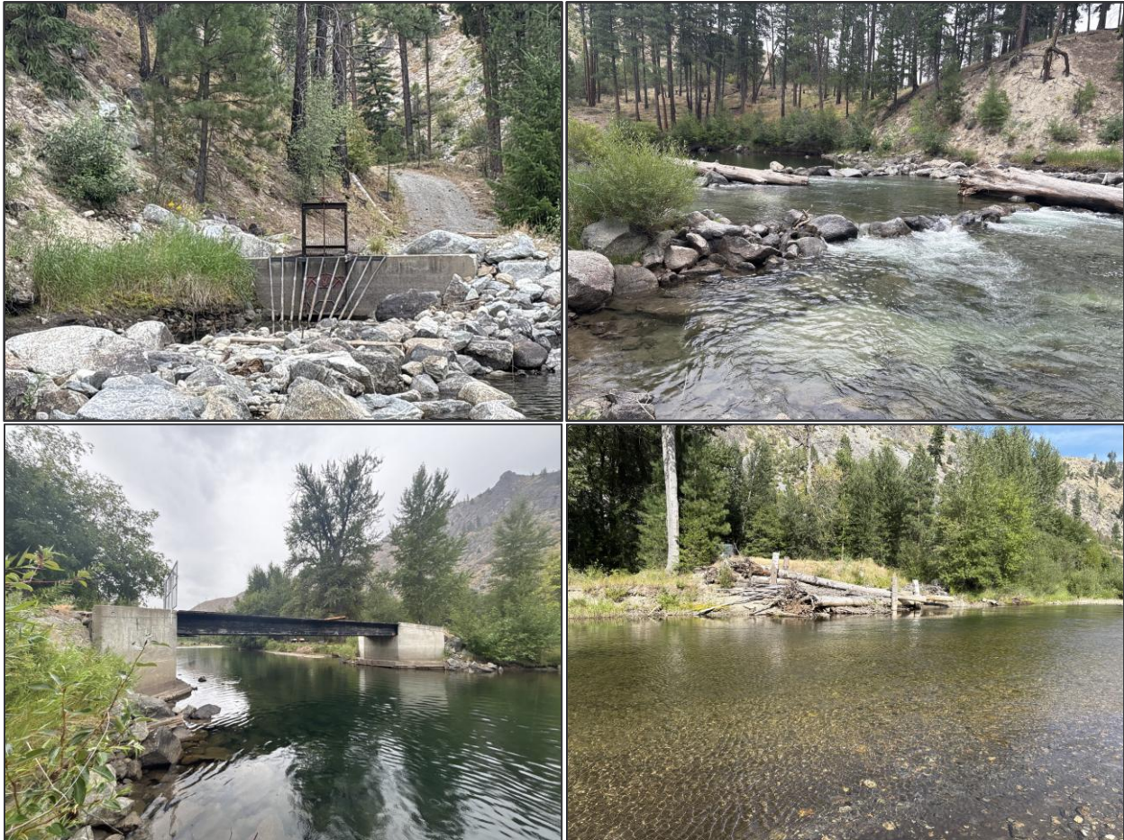
Figure 24. Human alterations in Segment 1. Top left: McKenzie Ditch (RM 16.6); Top right: boulder weirs directing flow into McKenzie Ditch, looking upstream; Bottom left: bridge and associated riprap at RM 18.1, looking downstream; Bottom right: fill associated with former Cottonwood Flats bridge (RM 18.45).
