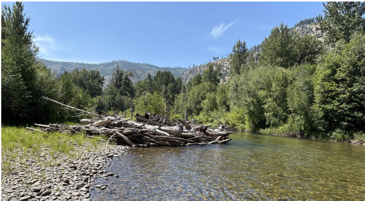
Figure 52. Stormy B constructed large wood structure at RM 20.8 looking downstream. Structure provides cover and deflects flows toward river right bank.
