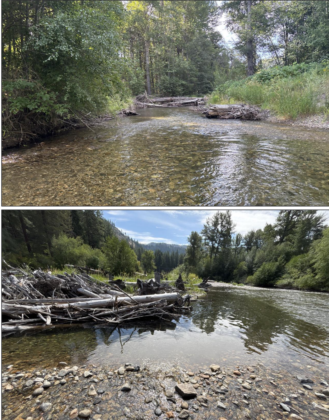
Figure 53. Representative photographs of Stormy A restoration project. Top: constructed side channel looking downstream from the upstream end. Bottom: constructed large wood structure providing cover on river left at RM 21.35.
