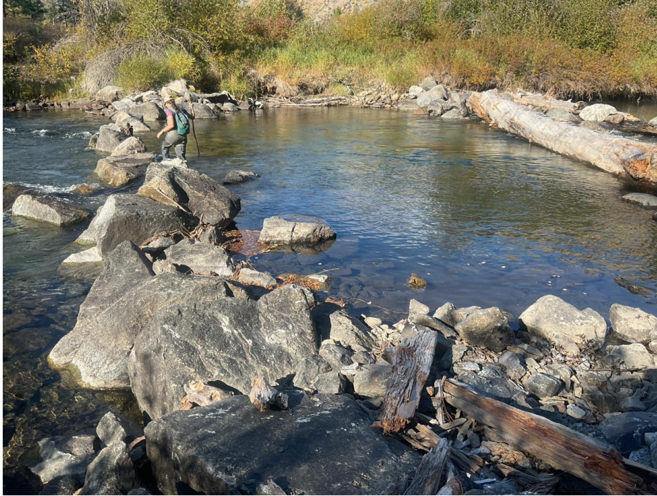
Figure 13. Photo shows the channel spanning rock weirs, adjacent to the McKenzie Ditch Irrigation Diversion near RM 16.65, forming pool habitat.
