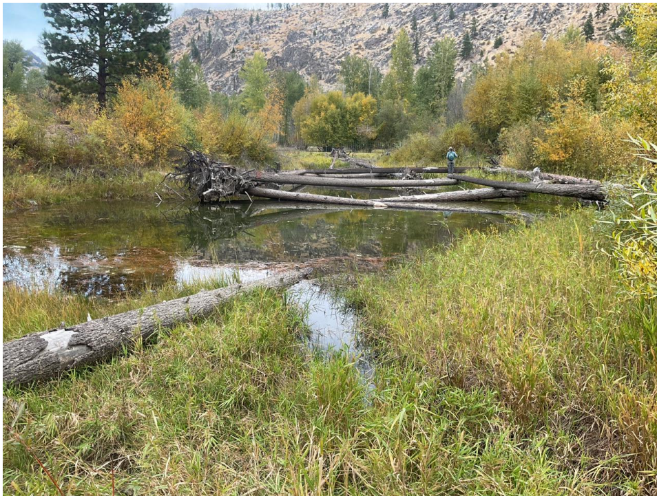
Figure 20. Alcove near RM 17.70, with placed LWM.
