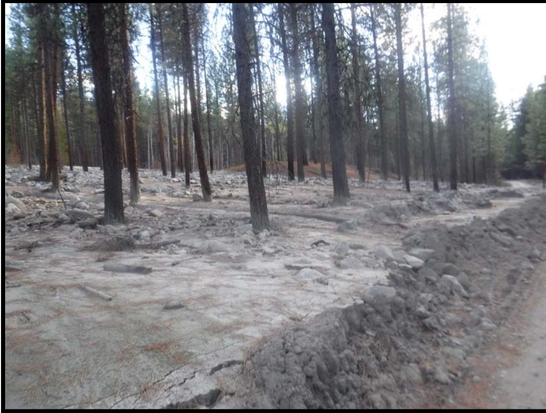
Figure 4. Leroy Creek debris flow runout taken along the East Chewuch Road.
