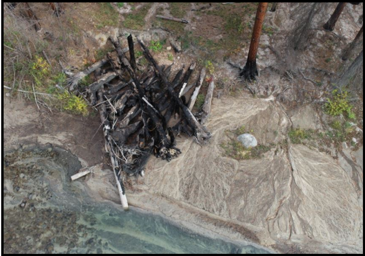
Figure 6. Photo showing typical mainstem large wood structure burn and post fire burial from 2022 Leroy Creek debris flow.
