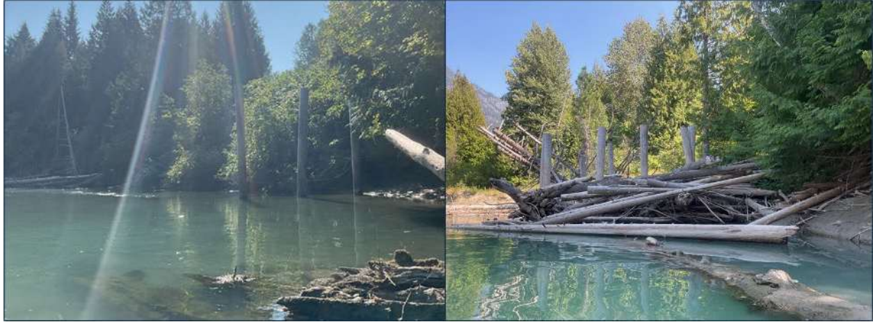
Figure 71. Left: Example of constructed wood piling structure with no effective function at RM 2.73 (August 15, 2024). Right: constructed wood piling structure effectively accumulating and retaining large wood at RM 3.32 (August 14, 2024).
