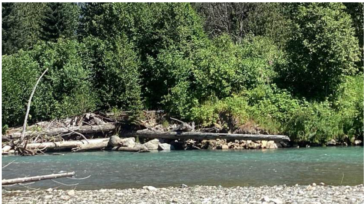
Figure 163. Riprap and large wood constructed bank protection along White River Road at RM 12.92 (August 4, 2024).
