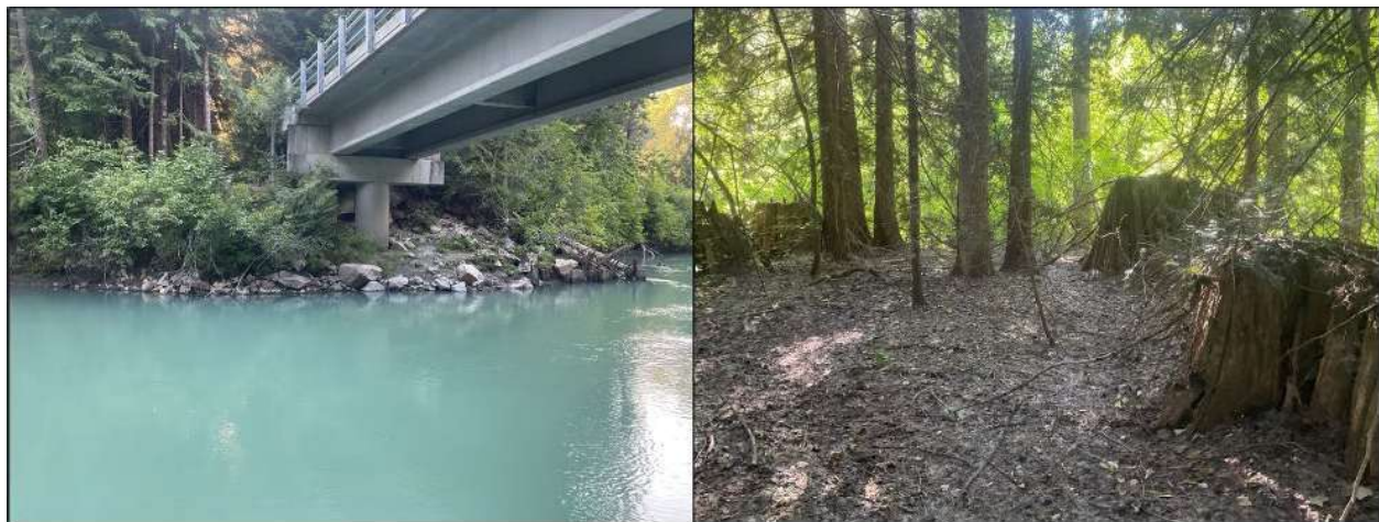
Figure 105. Left: Sears Creek Bridge and associated bank protection at RM 7, upstream Reach 4 boundary (August 6, 2024). Right: Stumps on old growth western redcedar on river-right floodplain at RM 6.92 (August 12, 2024).
