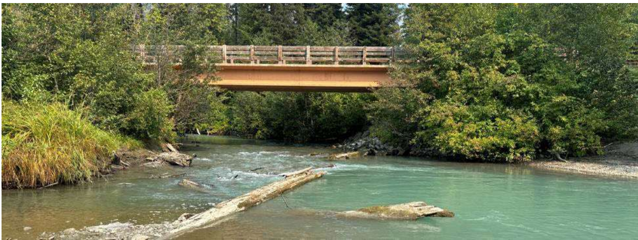
Figure 138. Bridge over the mouth of the Napeequa River at its confluence with the White River at RM 12.43, at upstream boundary of Reach 7 (September 7, 2024).
