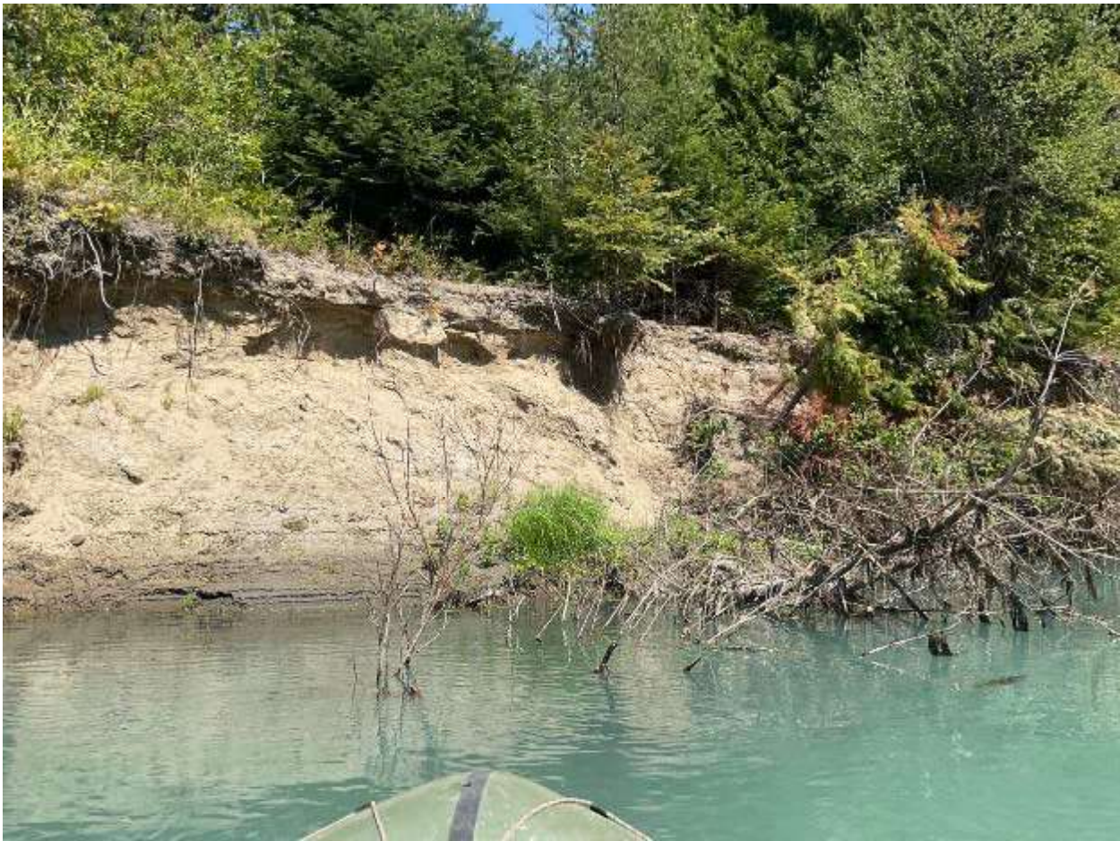
Figure 68. Exposed cut bank at RM 3.82, on river right. (August 14, 2024)
