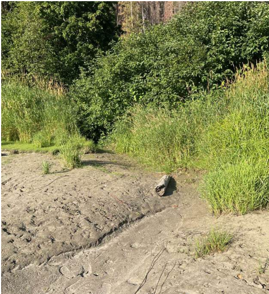
Figure 81. Outlet of dry tributary entering from river right just downstream of RM 4.7 (August 14, 2024).
