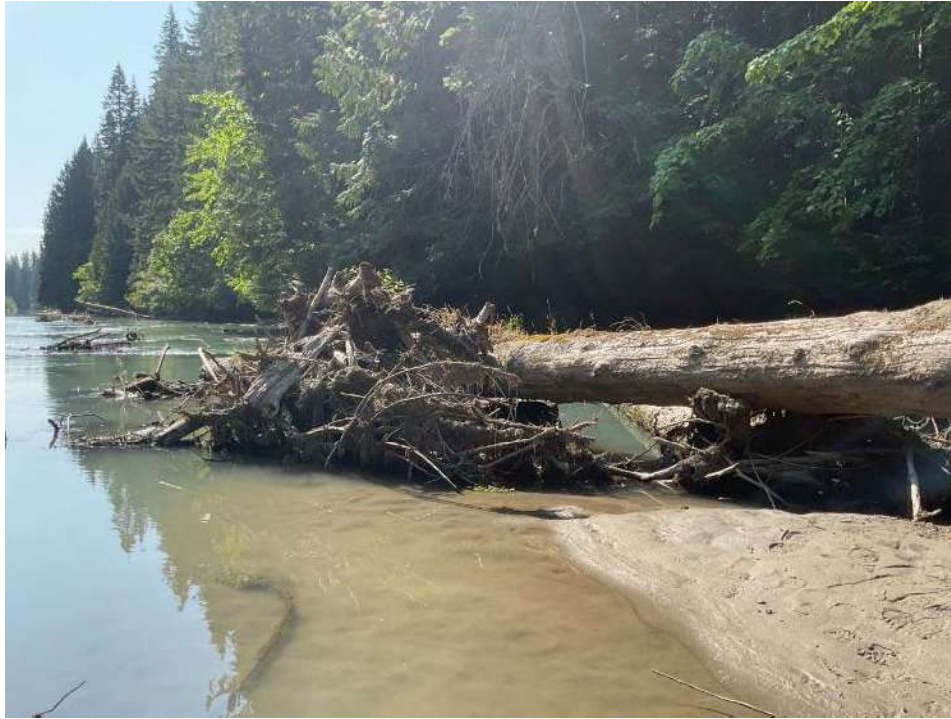
Figure 100. Large wood accumulation with alcove and localized scour at RM 6.35, looking downstream (August 13, 2024).
