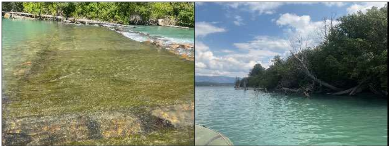
Figure 60. Left: Channel-spanning weir of rock and wood at RM 1.65, viewed from river right. (August 15, 2024) Right: Constructed large wood pilings at RM 0.06, looking downstream (August 16, 2024).
