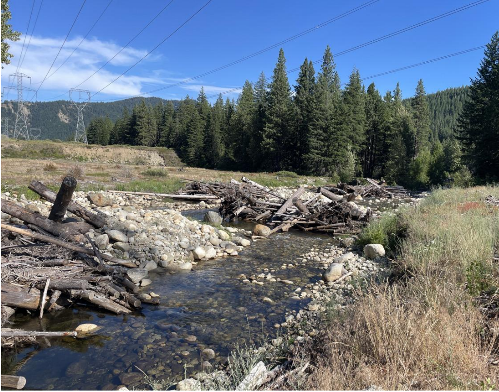
Figure 108. Constructed large wood structures in river-right side-channel near RM 6.6.
