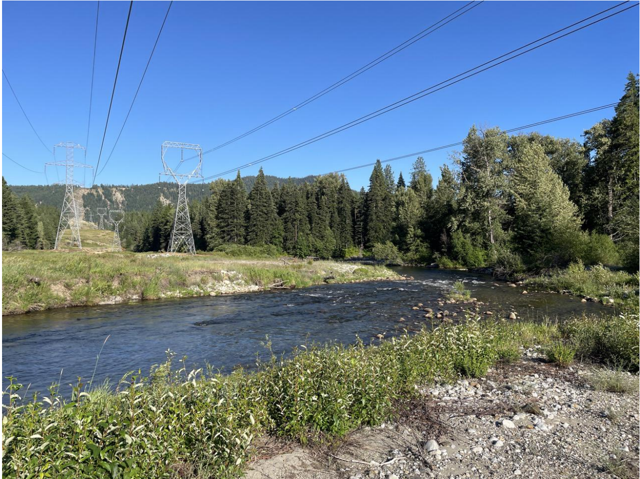
Figure 83. View looking downstream near RM 5.9 at area of channel with denuded riparian vegetation within the BPA powerline corridor (Inter-Fluve photo July 2025).
