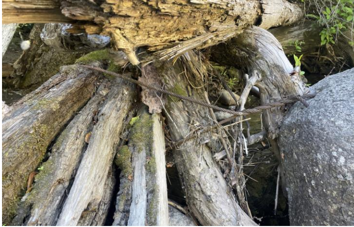
Figure 32. Log cabled to a boulder near RM 0.75.
