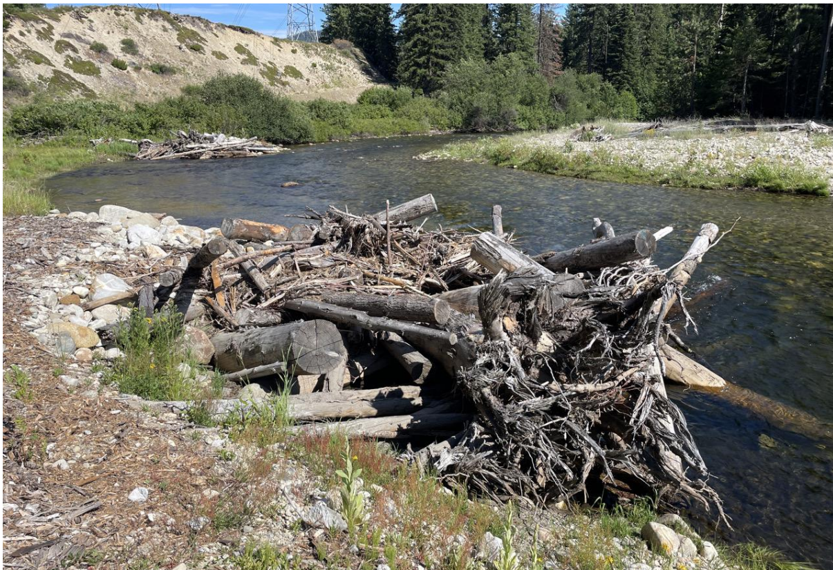
Figure 99. Constructed large wood structures near RM 7.1.
