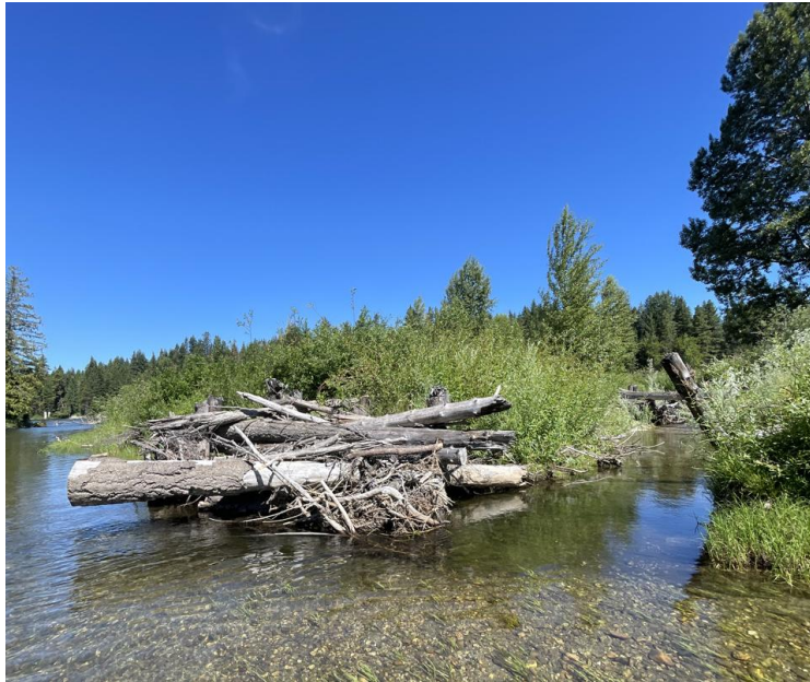
Figure 38. Inlet of constructed side-channel and wood placements on river-right as part of Nason Confluence Project near RM 0.1.
