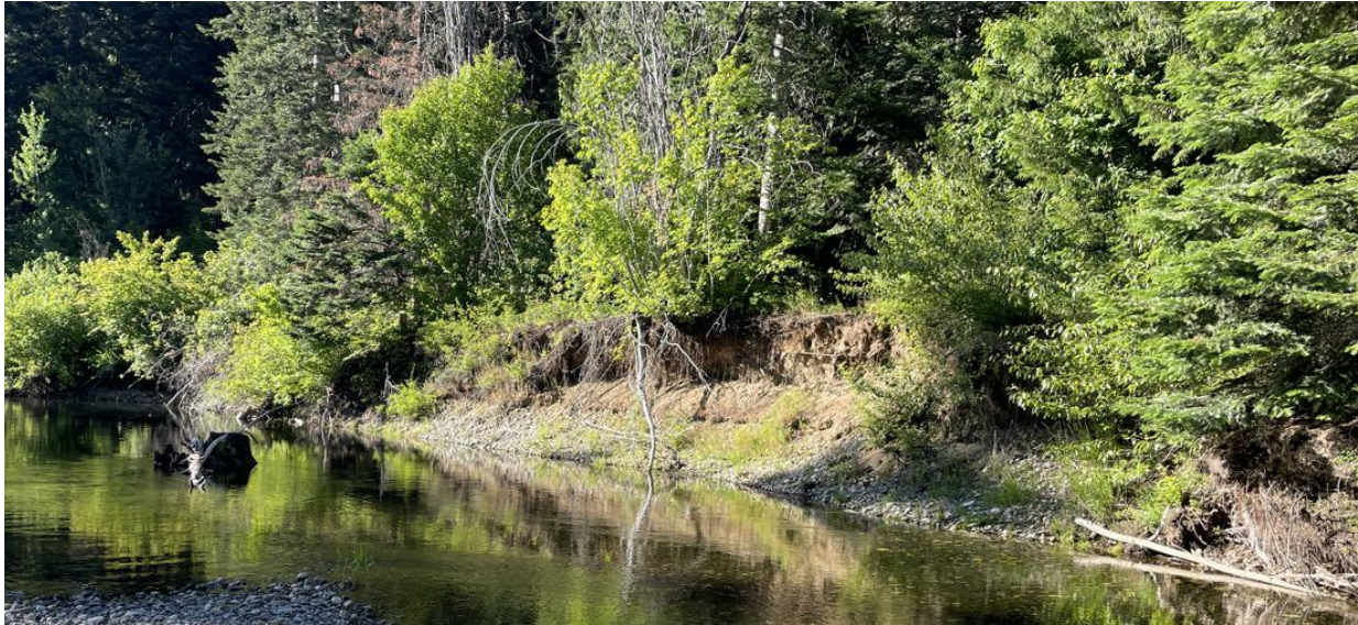
Figure 117. View upstream at eroding river-left bank near RM 11.2 (Inter-Fluve photo June 2025).
