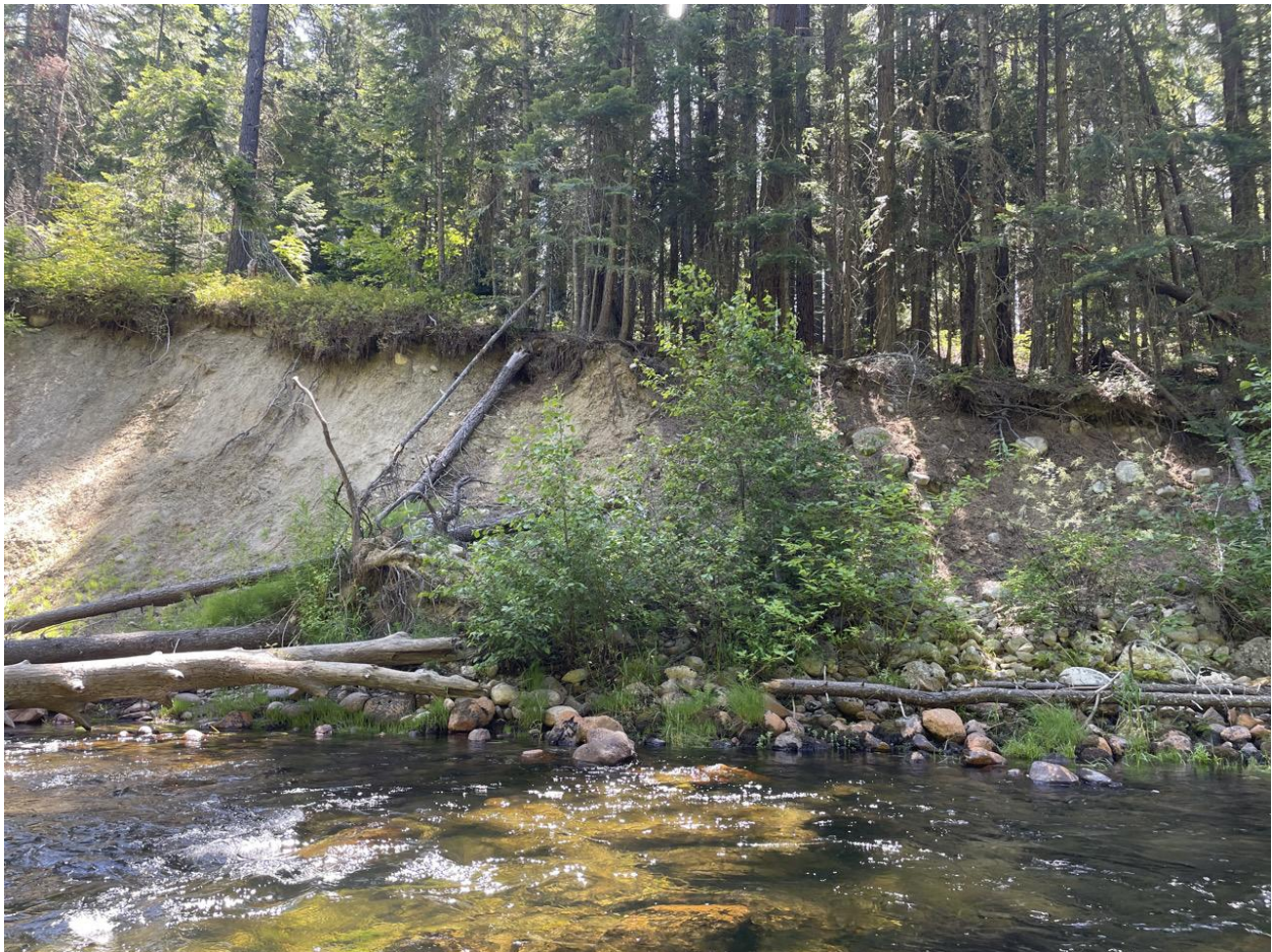
Figure 92. Boulders sourced from river-right bank near RM 8.8.
