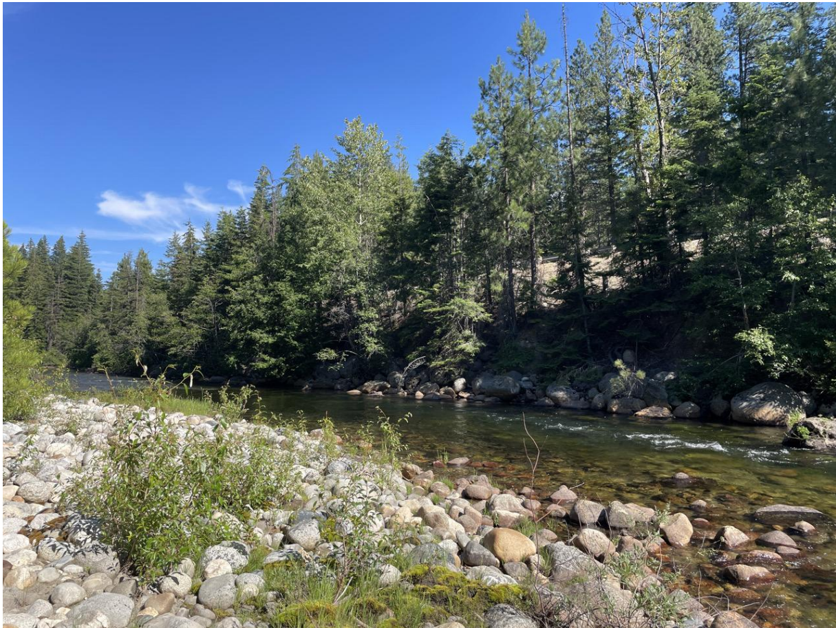
Figure 91. View downstream at riprap along the road fill on river-right near RM 6.9.
