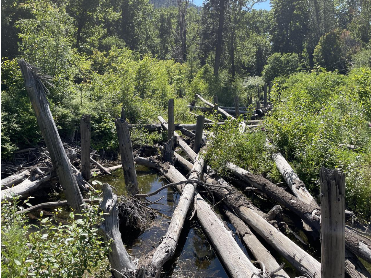
Figure 152. Constructed alcove with large wood placements near RM 12.1 (Inter-Fluve photo June 2025).
