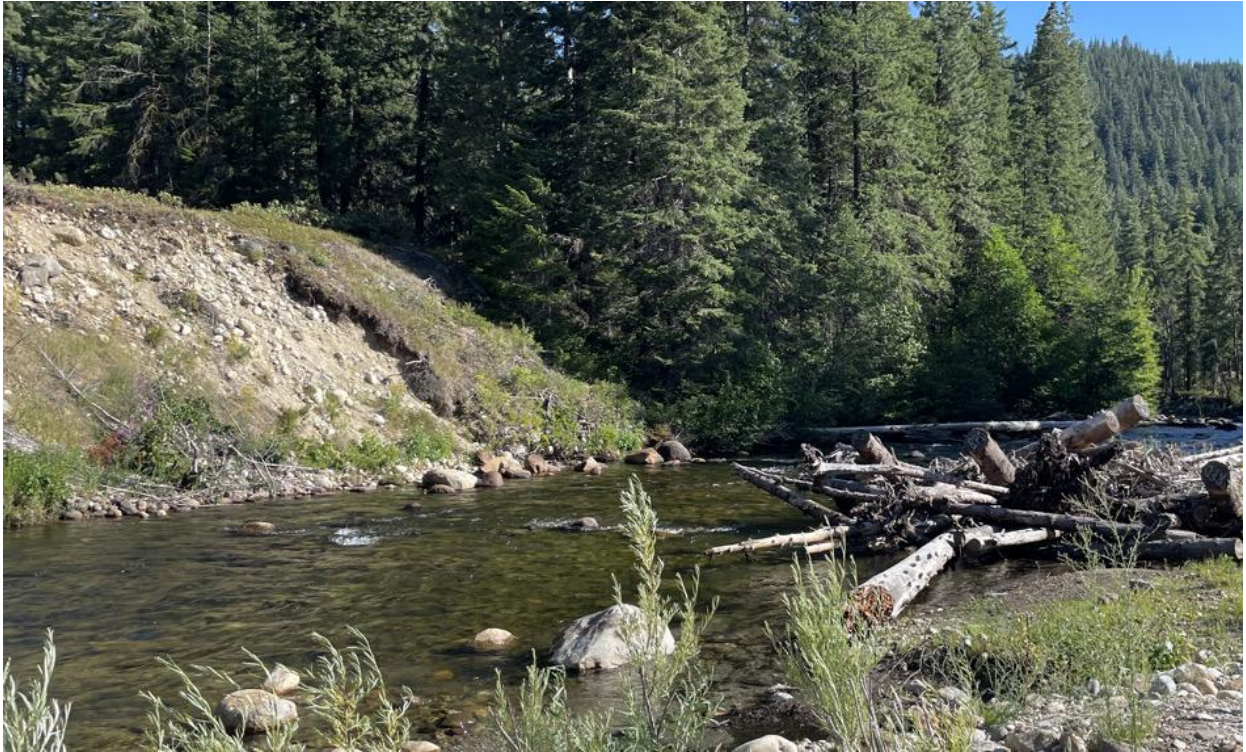
Figure 93. View downstream near RM 6.5 where the river is eroding into glacial deposits on the river-left bank.
