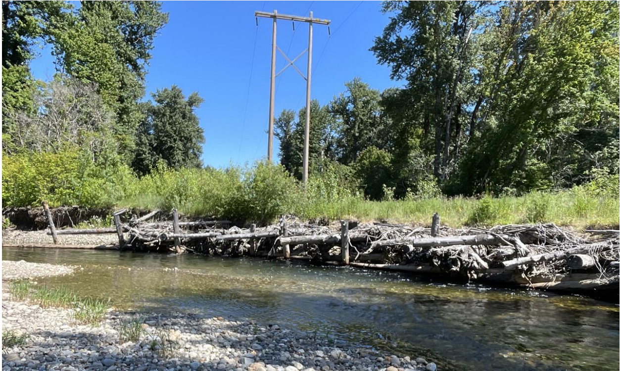
Figure 151. View downstream of 'powerline bend' jam at RM 12.45. Some erosion can be seen at the downstream portion of the jam (Inter-Fluve photo June 2025).
