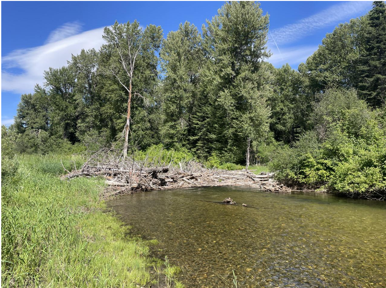
Figure 65. Channel-spanning jam at RM 2.25. Aerial photos suggest that this Jam was originally constructed as a left-bank jam that collected additional wood and became channel-spanning. The jam is very effective at keeping the right-bank side-channel active. The inlet is at the right side of the jam in the photo (Inter-Fluve photo July 2025).
