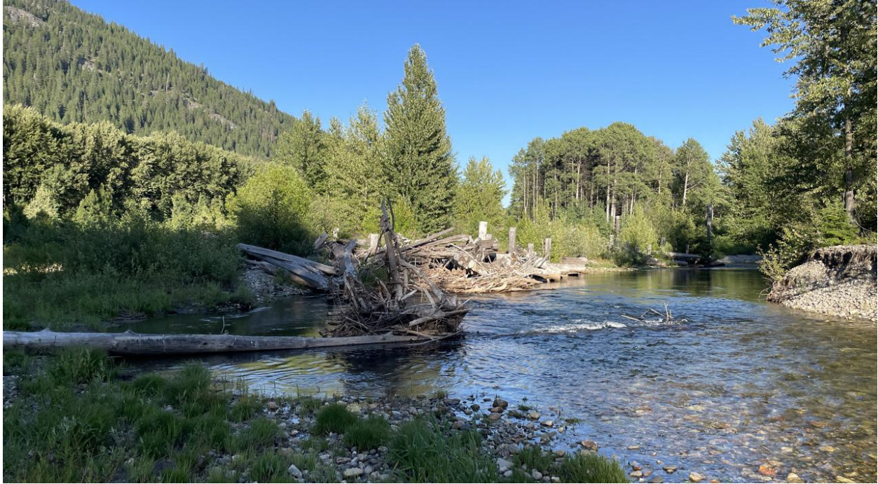
Figure 126. View downstream into cut-off channel at First Bend project site. Photo taken from RM 10.8 (Inter-Fluve photo June 2025).
