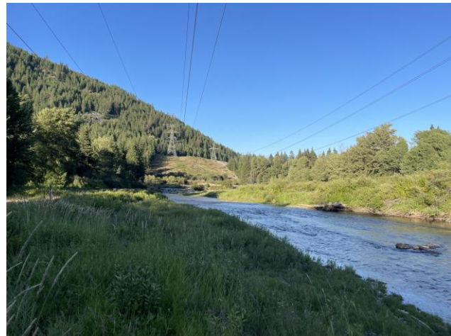
Figure 112. View downstream near RM 10.2 showing highly impacted channel and riparian conditions within the BPA powerline corridor (Inter-Fluve photo June 2025).
