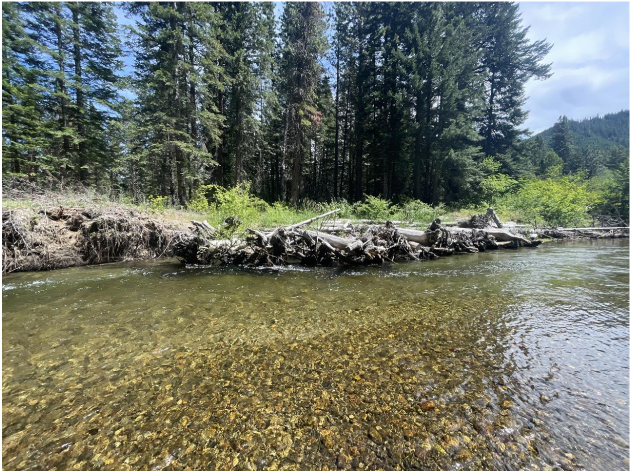
Figure 106. Nason Kahler project constructed log jam near RM 8.35.
