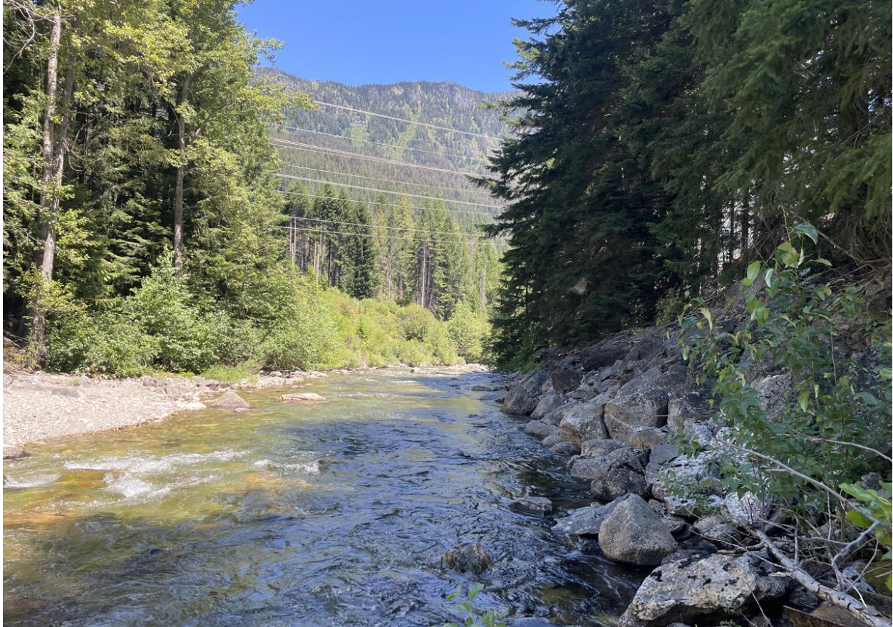
Figure 141. View downstream near RM 13.8. Riprap from the railroad embankment can be seen on river-right and bed material sourced from the Mahar Creek alluvial fan can be seen on river-left. BPA powerline crossing and related vegetation impacts can be seen in the background on river-left.
