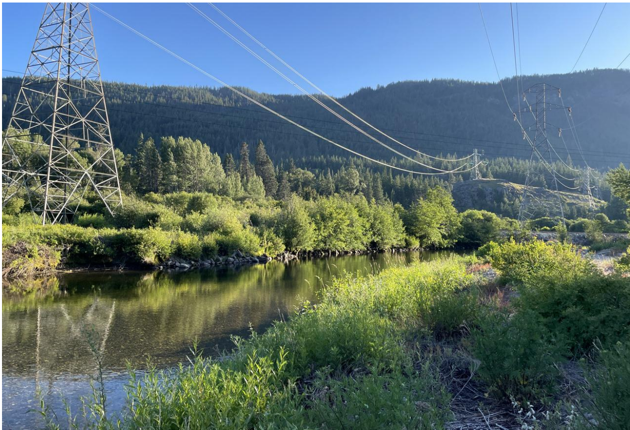
Figure 122. Example of complete loss of large wood recruitment potential due to bank armoring and clearing under the BPA powerlines. View upstream near RM 10.2.
