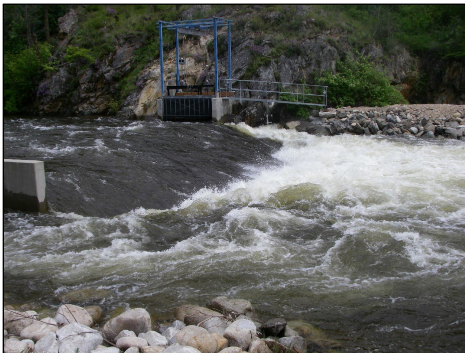
Figure 3.2.3. Chewuch Dam at high flow, June 2010. The fish passage channel can be seen to left of concrete wall at left side of image.
