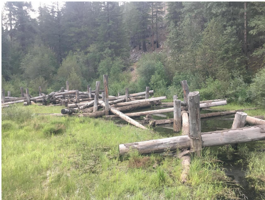
Figure 9. CWP #061, Chewuch - Doe AU, 22 August 2022. Large wood was installed in this springbrook wetland complex for cover and complexity in the Chewuch RM 11-13 project in 2013. Coho salmon parr were observed in this CWP during the site visit in 2022.
