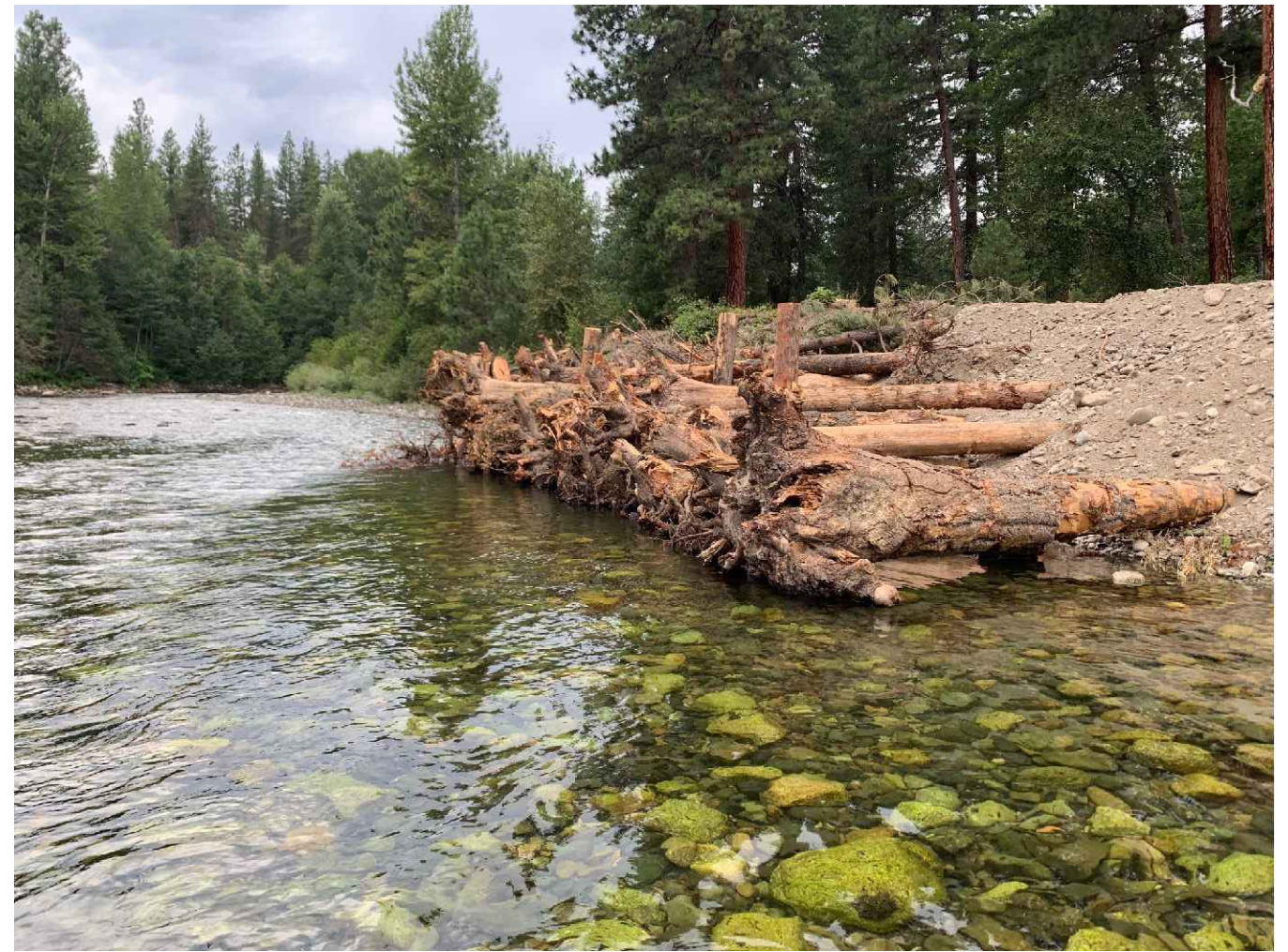
TYPICAL CONSTRUCTED BANK-BURIED LARGE WOOD STRUCTURE
