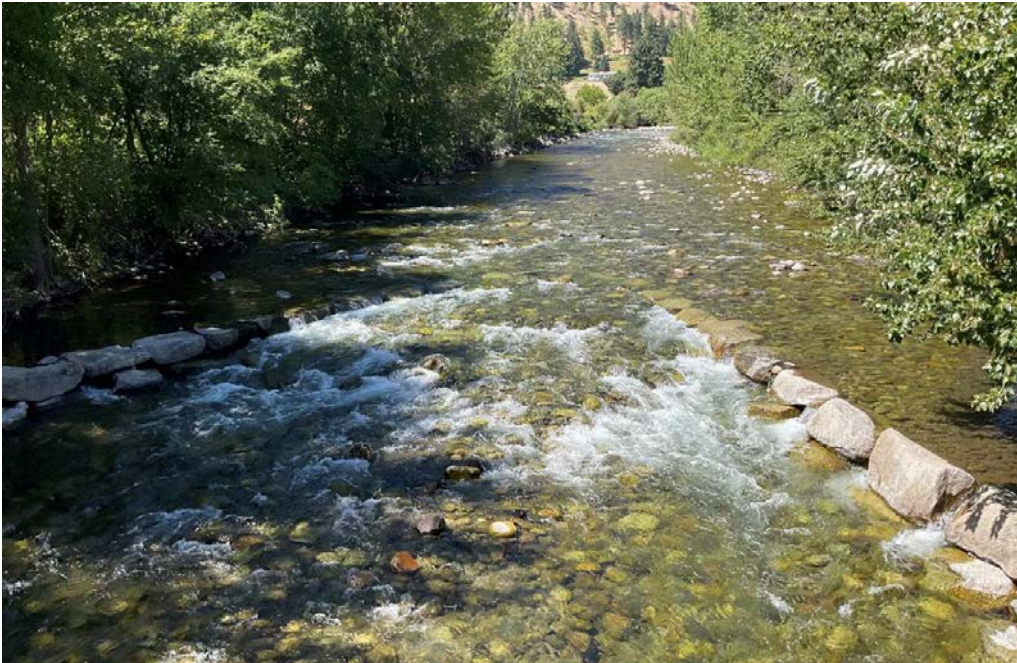
Figure 10: Downstream cross vane by Dinkelman Canyon Road bridge at RM 4.28
