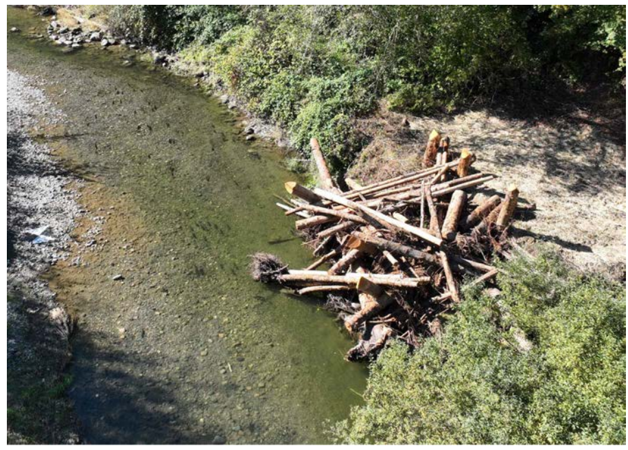
EXAMPLE OF COMPLETED DEFLECTOR ELJ
