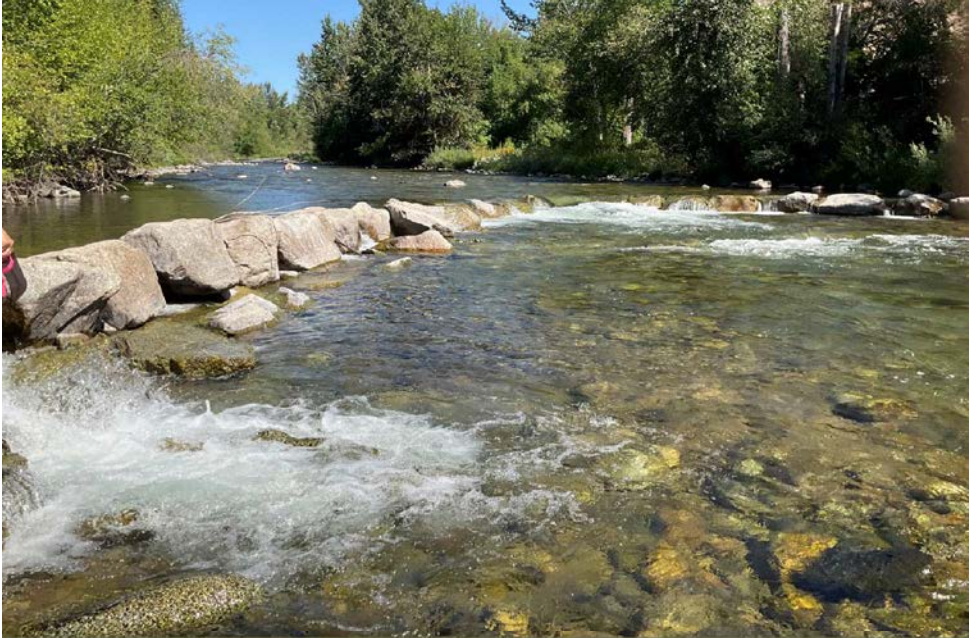
Figure 9: Upstream cross vane at Hanan-Detwiler diversion at RM 4.78.
