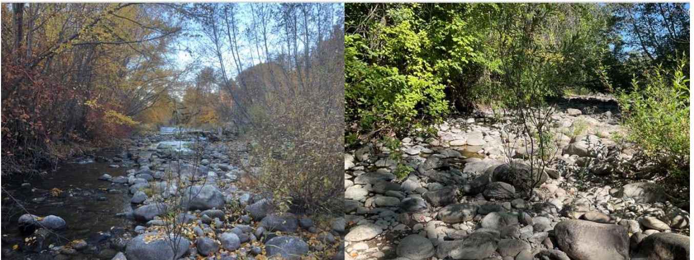
Figure 8: Seasonal side channel on river right at RM 4.73 below the Hanan-Detwiler cross vane. Left panel is November 2021 with shallow flow, right panel is dry in August 2023.
