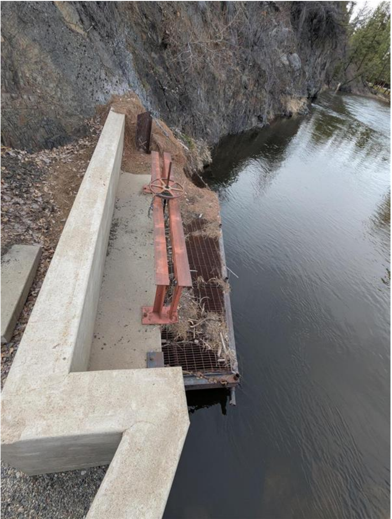
Trout Unlimited Inc.; Fulton Ditch Irrigation Efficiency Project Phase 2 (#25-1214)
