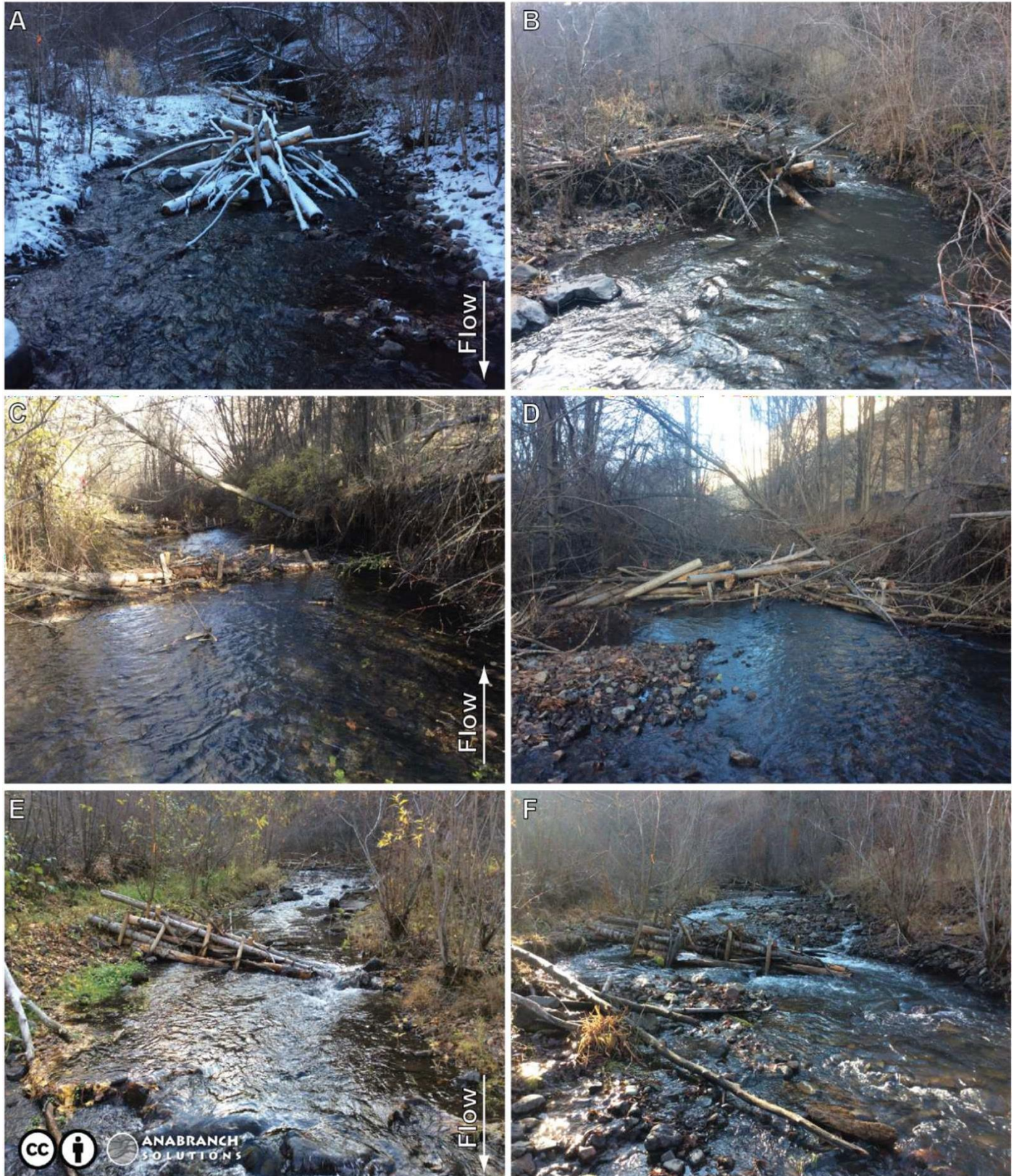
Figure 4. Example of PALS evolution over the course of one year promoting processes of wood accumulation. A and B show a mid-channel PALS becoming a bank-attached PALS, C and D show a bank-attached PALS becoming a debris jam, and E and F show a bank-attached PALS becoming a mid-channel PALS. The geomorphic changes imposed by the presence of the PALS in each example shows clear alterations to the channel bed and hydraulics. From Chapter 4 of Wheaton et al. (2019: http://lowtechpbr.restoration.usu.edu ).
