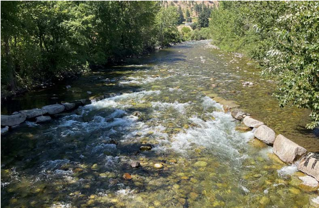
Figure 10: Downstream cross vane by Dinkelman Canyon Road bridge at RM 4.28
