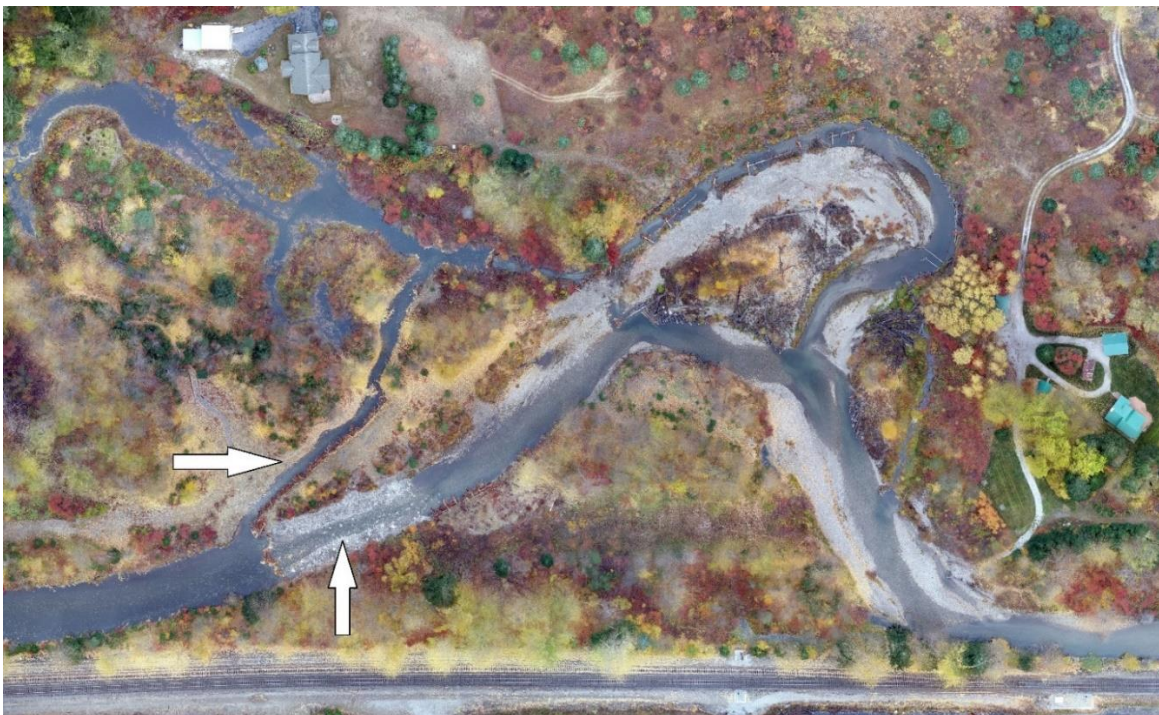
Photo: This aerial photo displays the Merritt Oxbow worksite, flowing left to right. The arrow on left (facing right) points to the newly created perennial side channel that connects to the pre-existing oxbow. The arrow on the bottom (facing up) points to the constructed riffle site shown in the top photo.
