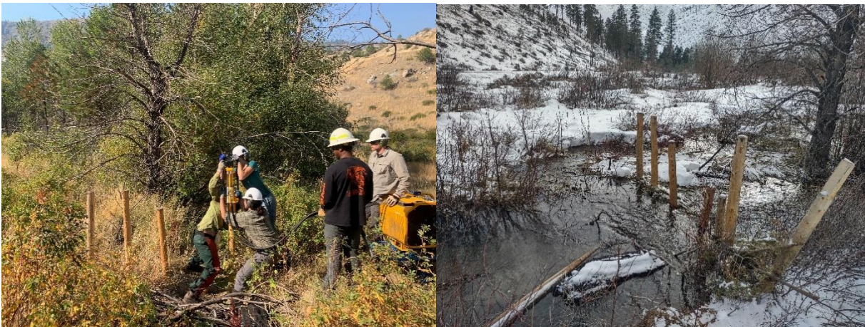
Photo: Cascadia CD, Trout Unlimited, Cascade Fisheries, and USFS staff install a series of 22 BDAs and PALS for Potato Creek in October of 2022. A look at the same BDA structure in February 2023 before freshet shows advanced floodplain inundation, stream bed aggradation, side channel activation, and channel widening.
