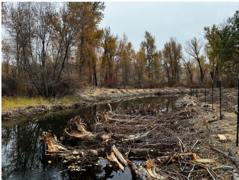
Photo: The new side channel post construction.
