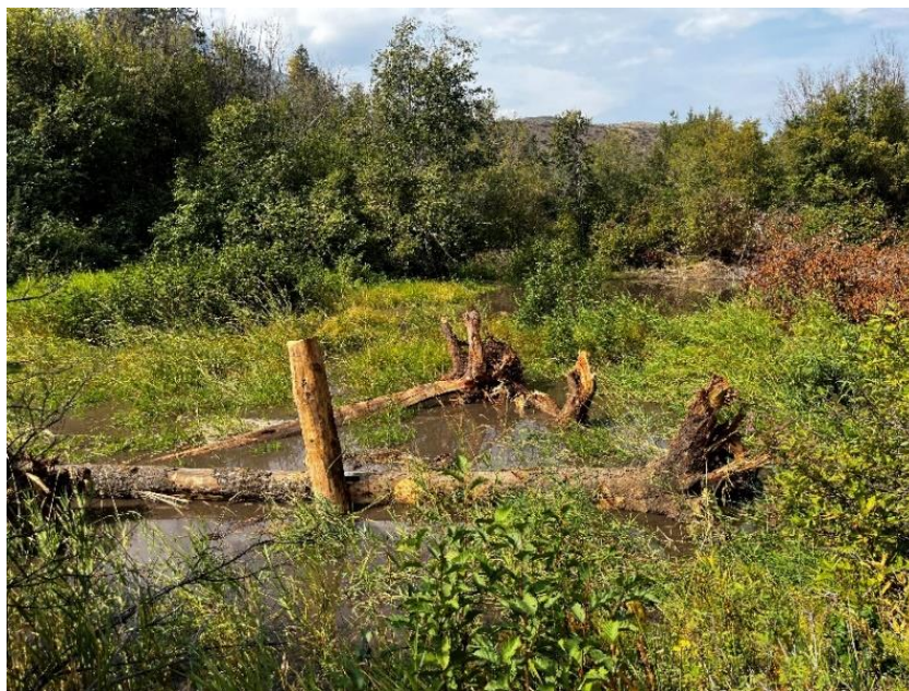
Photo: Engineered log jam immediately downstream of new side channel excavation.
