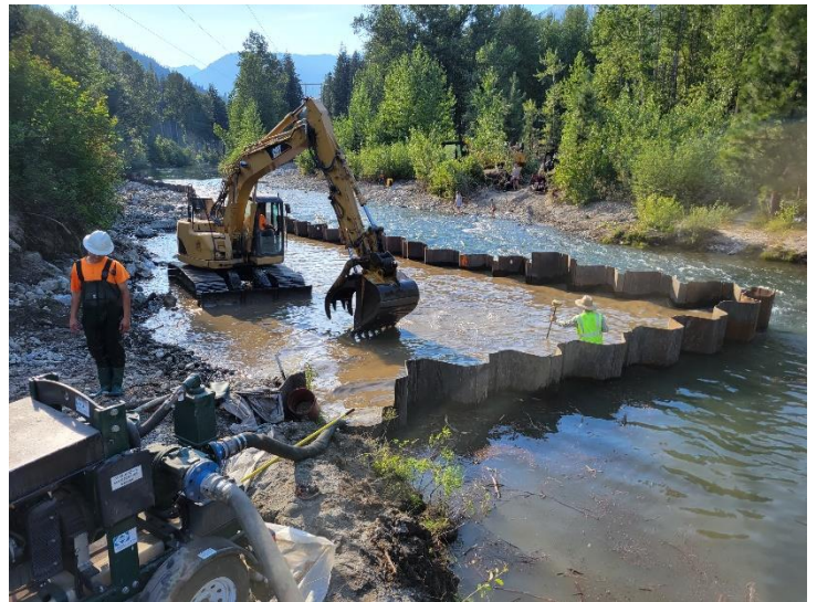
Photo: Use of heavy equipment is common in large-scale restoration projects. Here the contractor carefully works instream to build the constructed riffle, which increased the elevation of Nason Creek to ensure water flows through the newly created side channel.
