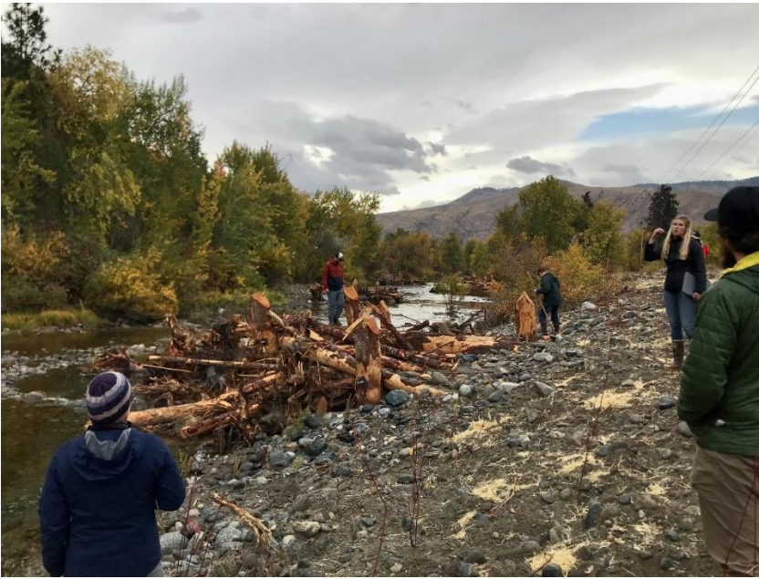
Chelan County Natural Resources staff lead a post-construction project tour in October 2021. Multiple engineered log jams can be seen on both banks of the side channel.
