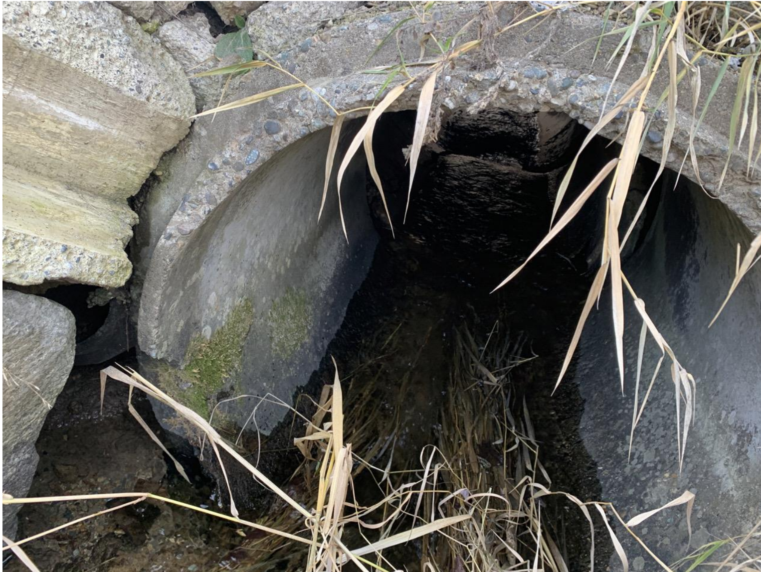
Chelan Co Natural Resource; Eagle Creek Lowest Four Barrier Corrections (#23-1278)
