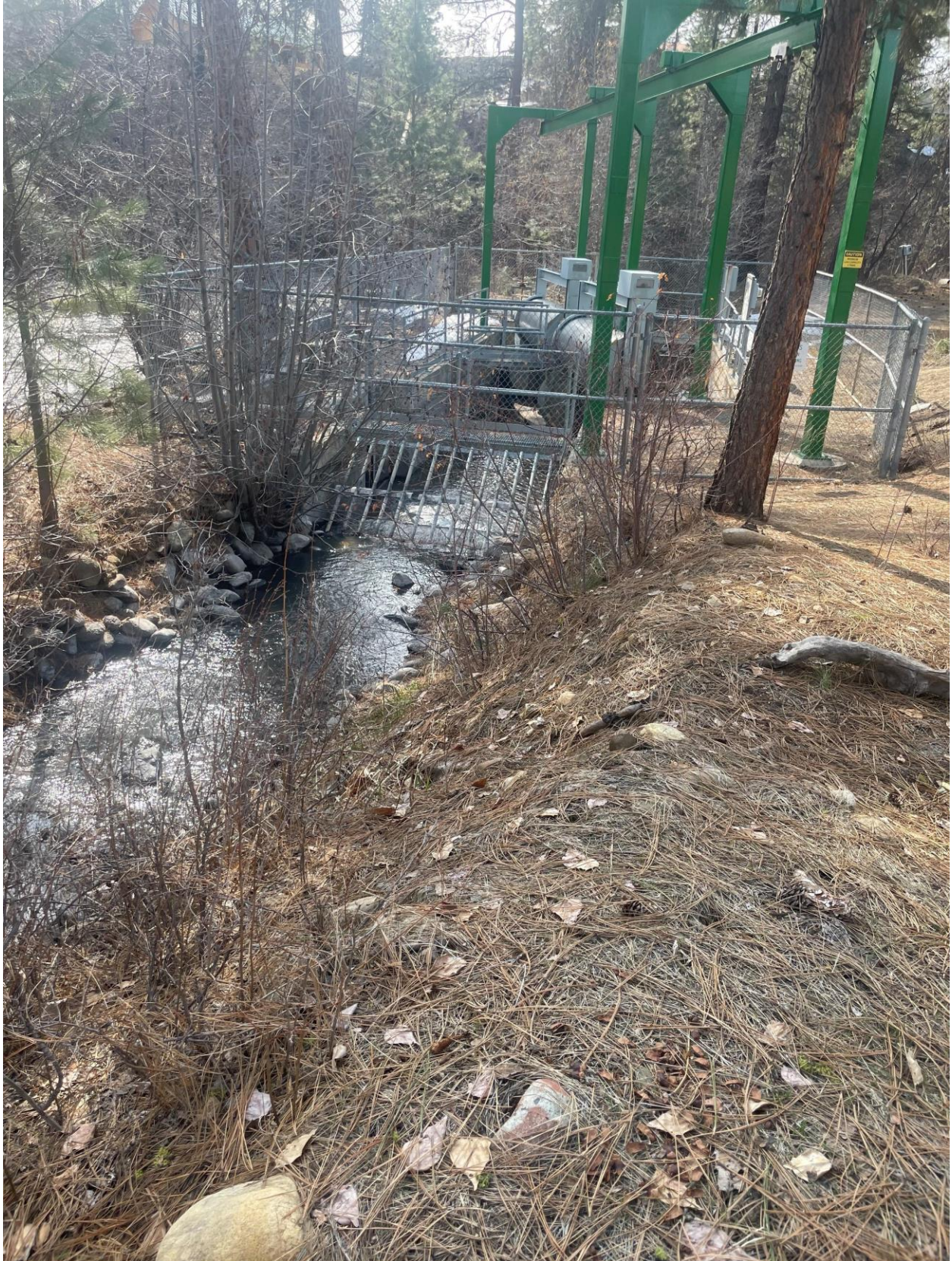
Trout Unlimited Inc.; Fulton Ditch Irrigation Efficiency Project Phase 1 (#23-1277)
