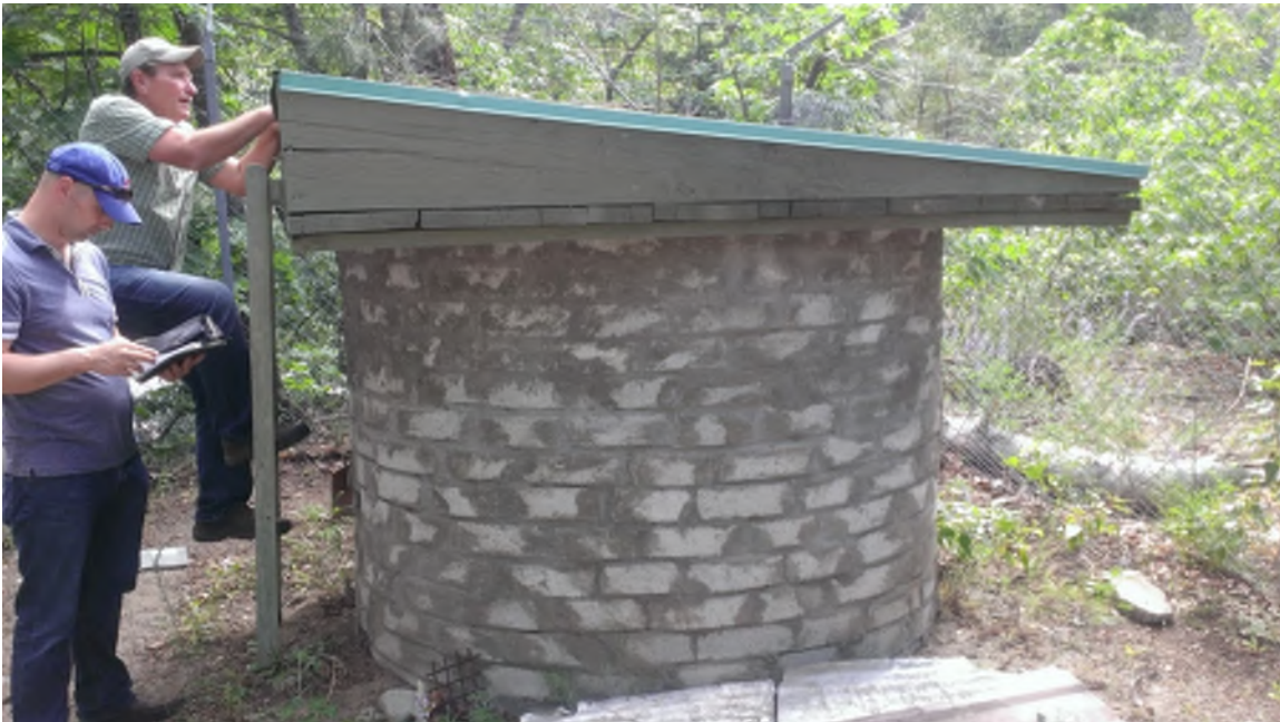
Photograph 4 Bifurcation, Valve Enclosure
