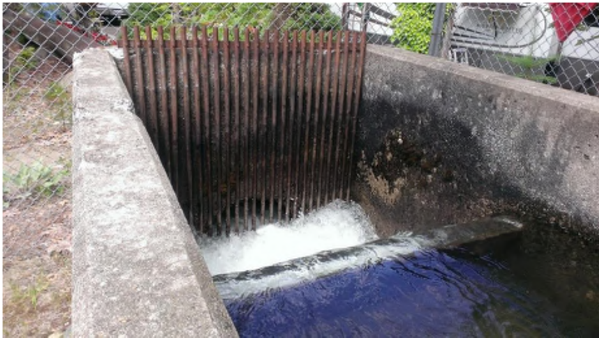
Photograph 8 Weir, Pipe Inlet, Debris Rack
