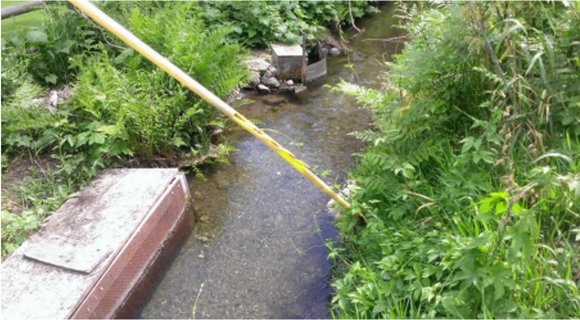
Photograph 15 Typical Turnout Structure West of Icicle Road
