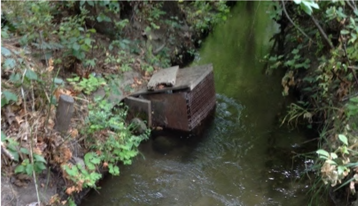
Photograph 17 Lateral Intake Structure West of Icicle Road
