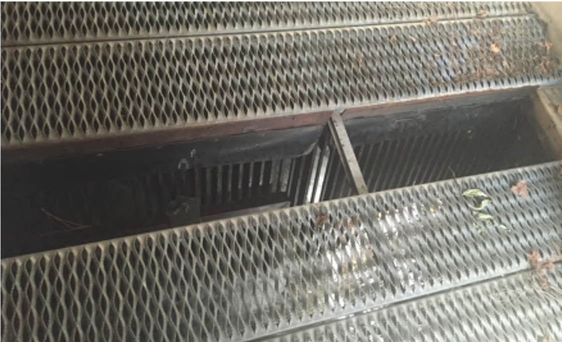
Photograph 2 Debris Rack at Inlet to Diversion Pipeline under Control House
