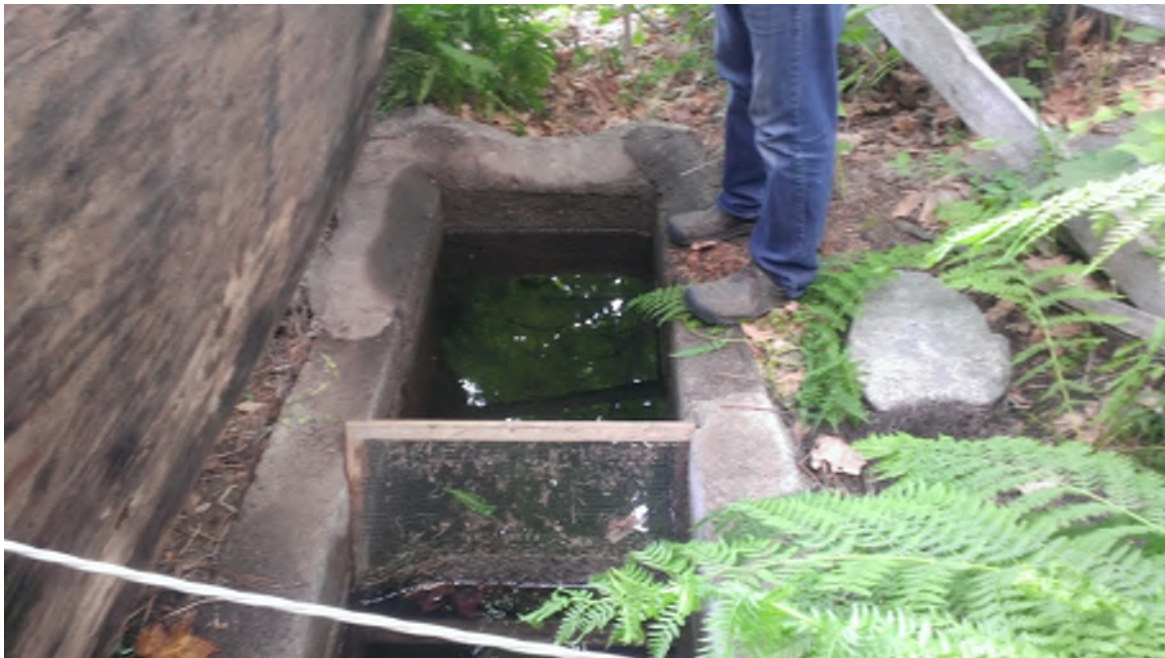
Photograph 18 Lateral Intake Structure West of Icicle Road
