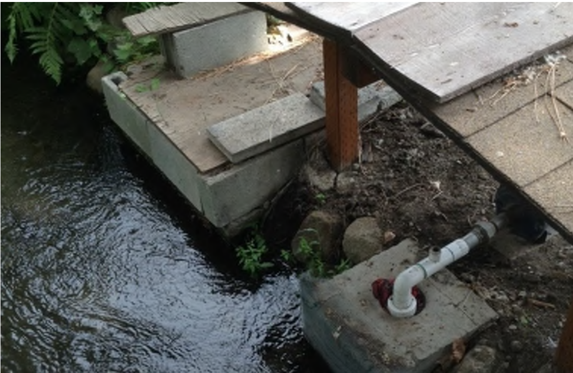
Photograph 16 Typical Pumped Turnout West of Icicle Road
