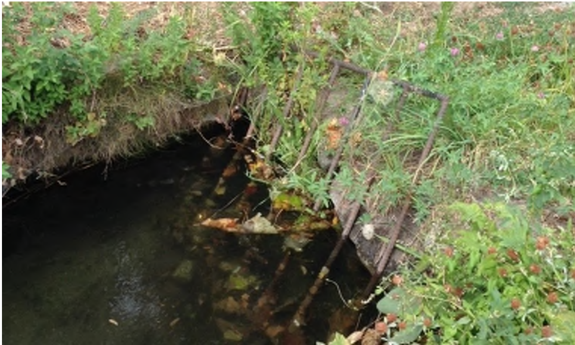
Photograph 14 Culvert Crossing at Shore Street
