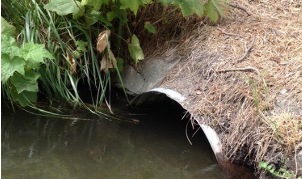
Photograph 13 Culvert Crossing at Icicle Road
