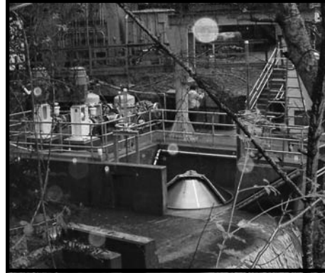
Above: Screen installed at shallow impoundment behind inflatable dam.
