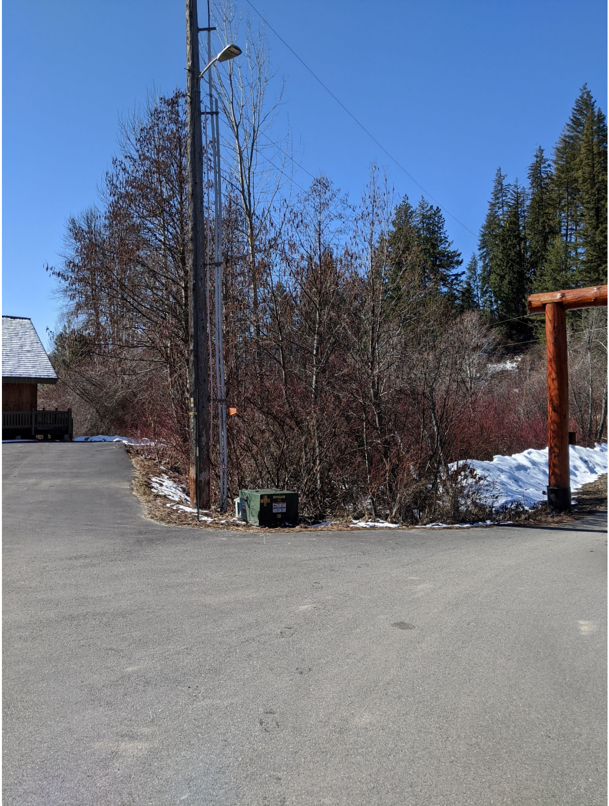
Photo 7. Looking downstream at utility pole and associated junction box near the existing culvert.
