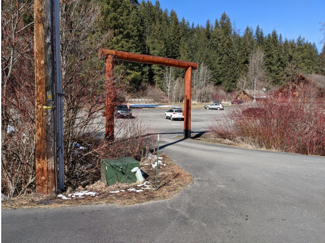
Photo 1. Looking west across existing culvert crossing.
